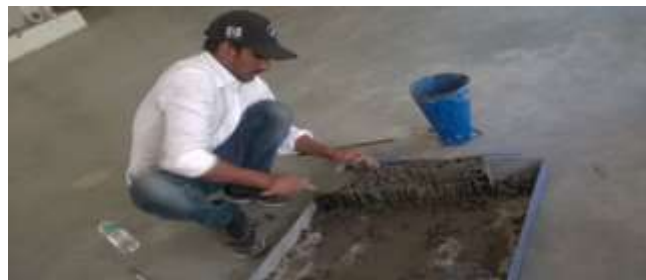
Fig. 1: Casting of Beam
